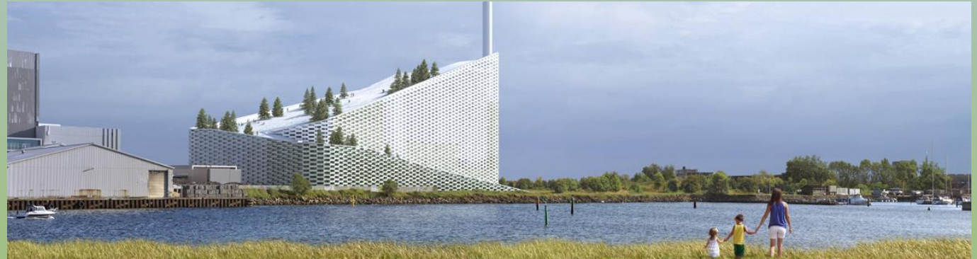
Biomass plant (woodchip) Copenhagen
